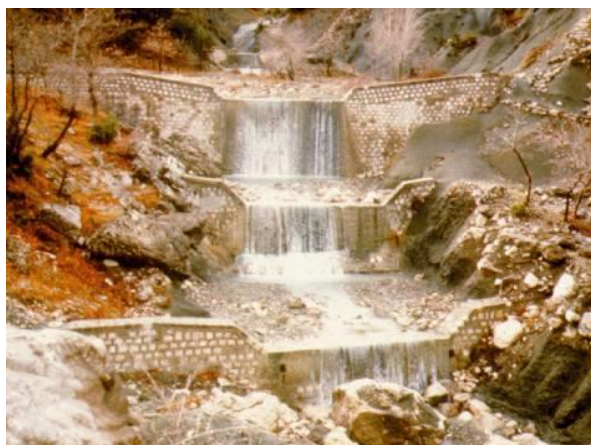
Dam for consolidation beds in the torrent of "Falls" in Pindos
