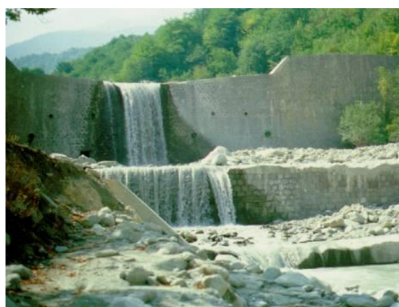
Dam for holding back the solid materials in the torrent of Orma (District of Aridea)
